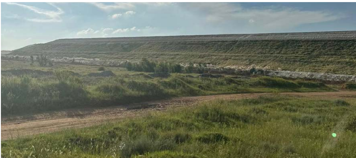
Figure 2. Rehabilitation of Doornkop tailings dam in Gauteng 16
