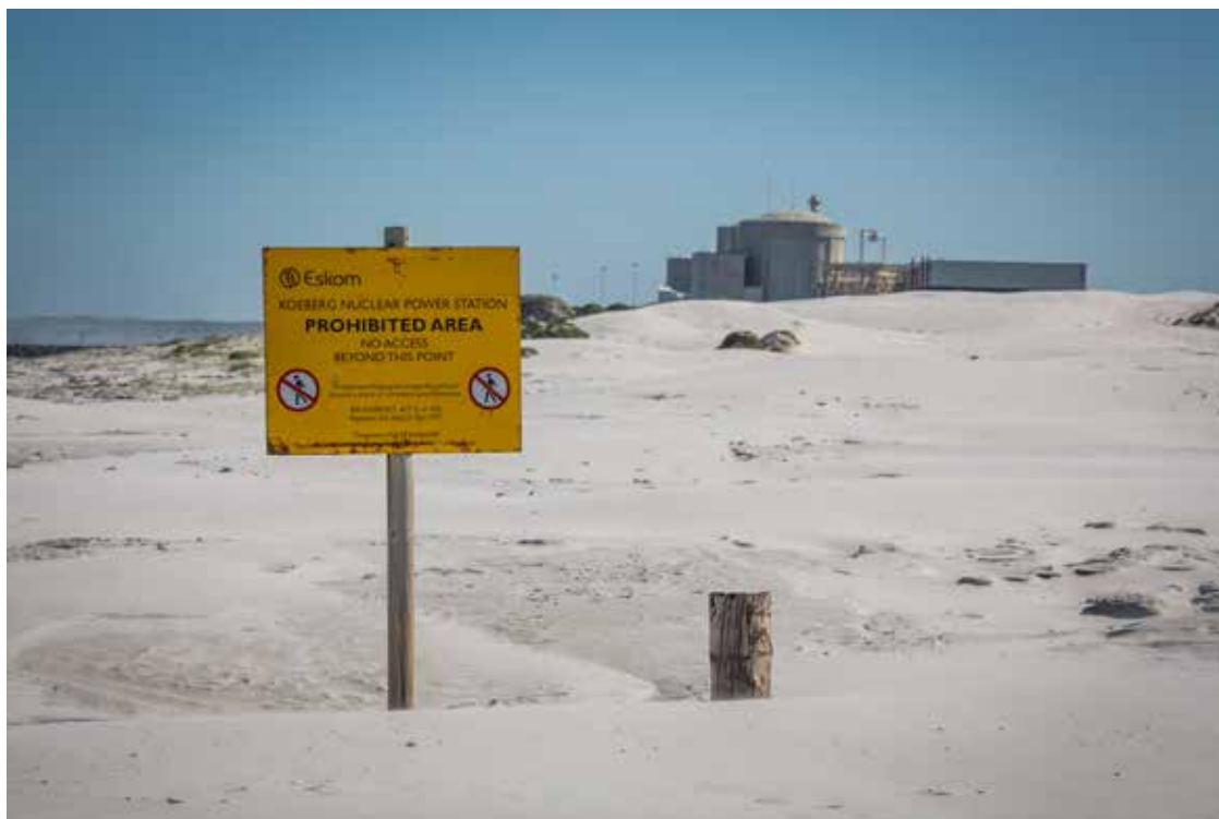
A view of Koeberg Power Station , Cape Town
